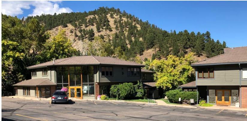
FIGURE 3 A NEW BUILDING RECONSTRUCTED AT SAME SITE
