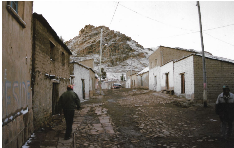
FIGURE 6 PROXIMITY TO MINES HELPED OCURÍ PRECOCIOUSLY DEVELOP ELECTRICITY
