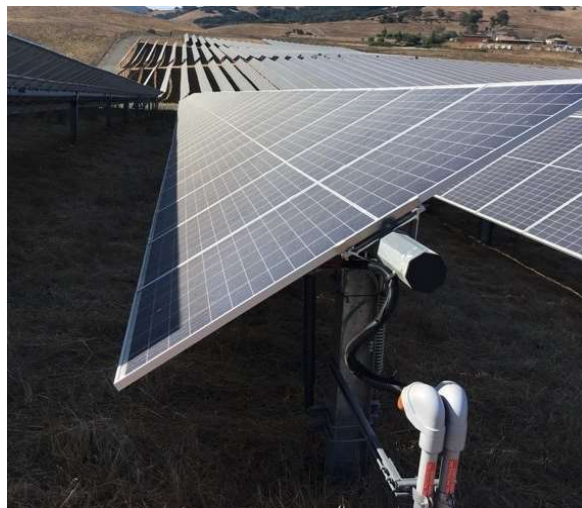
FIGURE 3 EVEN MINOR SHADING FROM ONE ROW TO THE NEXT DRAMATICALLY DECREASES OUTPUT
