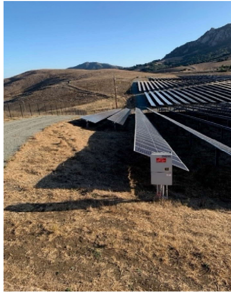
FIGURE 2 TOPOGRAPHY OF THE X SOLAR ARRAY SHOWING THE SKEWED NATURE OF THE SITE
