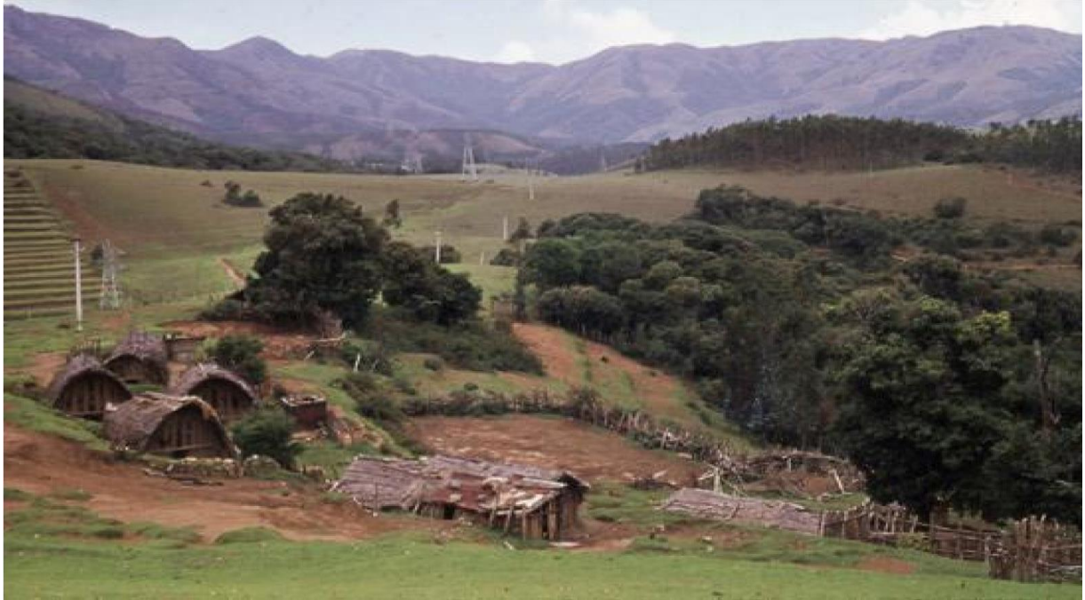
Figure 4. Distinctive Toda Architecture—1. Maintaining Tradition in the early 1970s: All four domestic dwellings retain the traditional barrel-vaulted structure; one set of calf sheds is located in the middle foreground, another downhill to the right; there are two large buffalo pens: one (circular) behind and downhill from the domestic area and the other (rectangular) downhill from the main calf shed cluster; a smaller circular pen for calves is downhill and to the right of the larger rectangular pen; recently installed electricity pylons reach to the hamlet's edge but, at the time (1974), were not yet bringing electricity to the hamlet. (Photo: Pauline H. Walker 1974, © Anthony R. Walker.)
